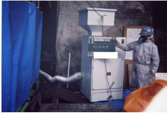
Fig. 13. Negative air pressure facility for removal of asbestos
