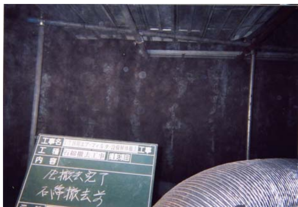
Fig. 11. Removal of asbestos in an air-heating furnace
