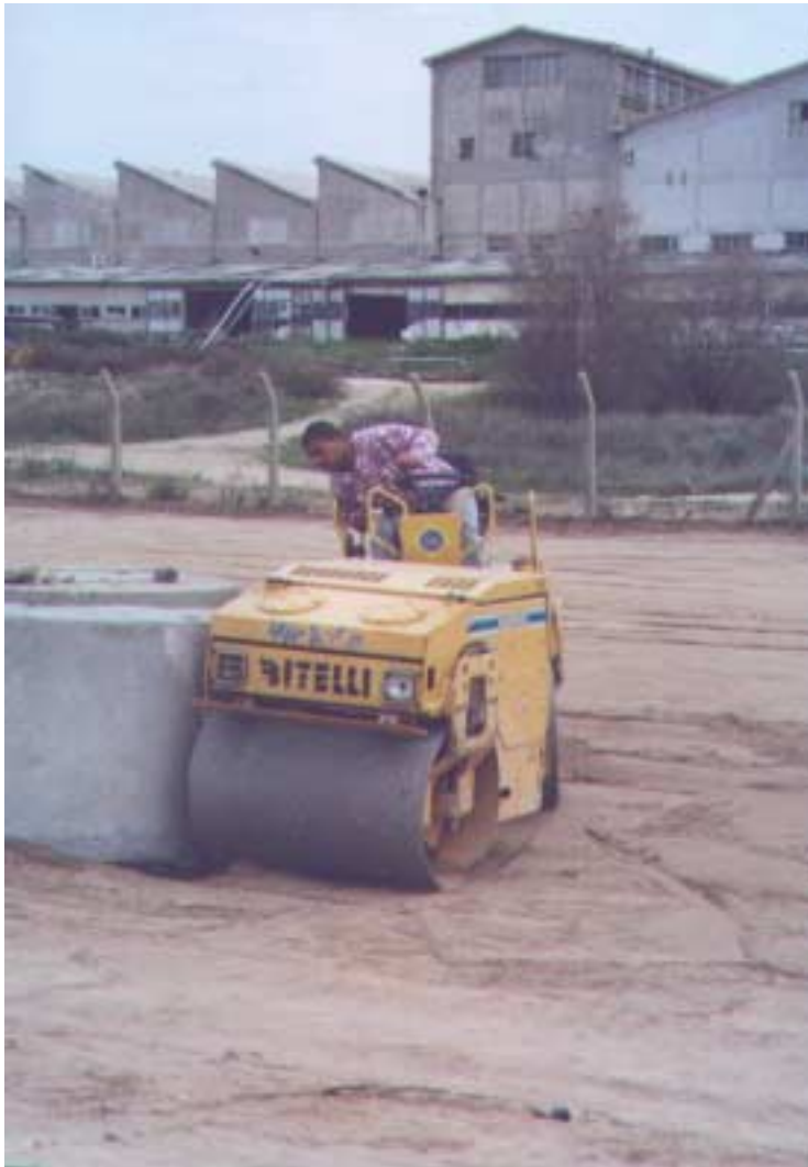
Figure 11. Packing dirt before installing protective membrane. [Full Size]
