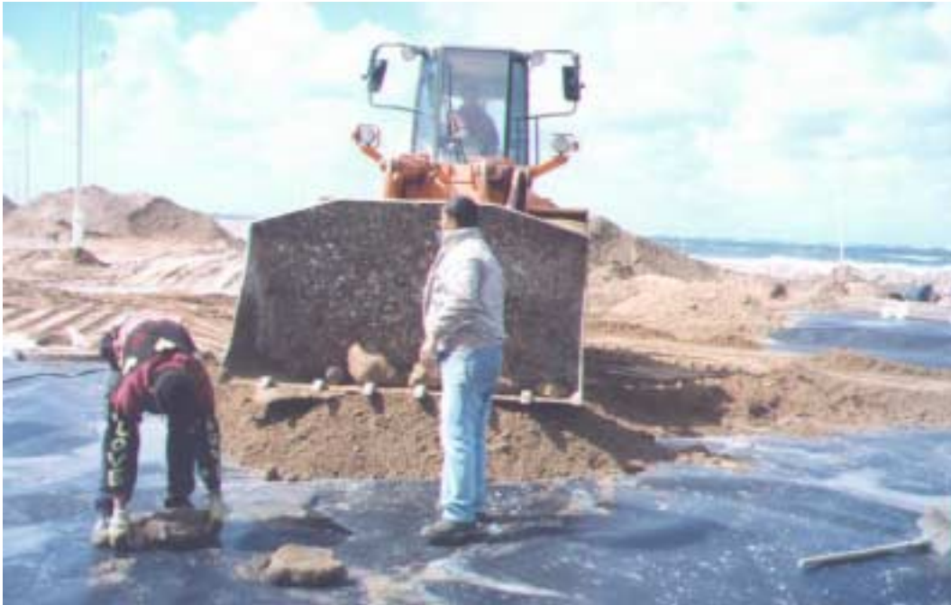
Figure 14. Covering geomembrane with clean fill dirt. [Full Size]
