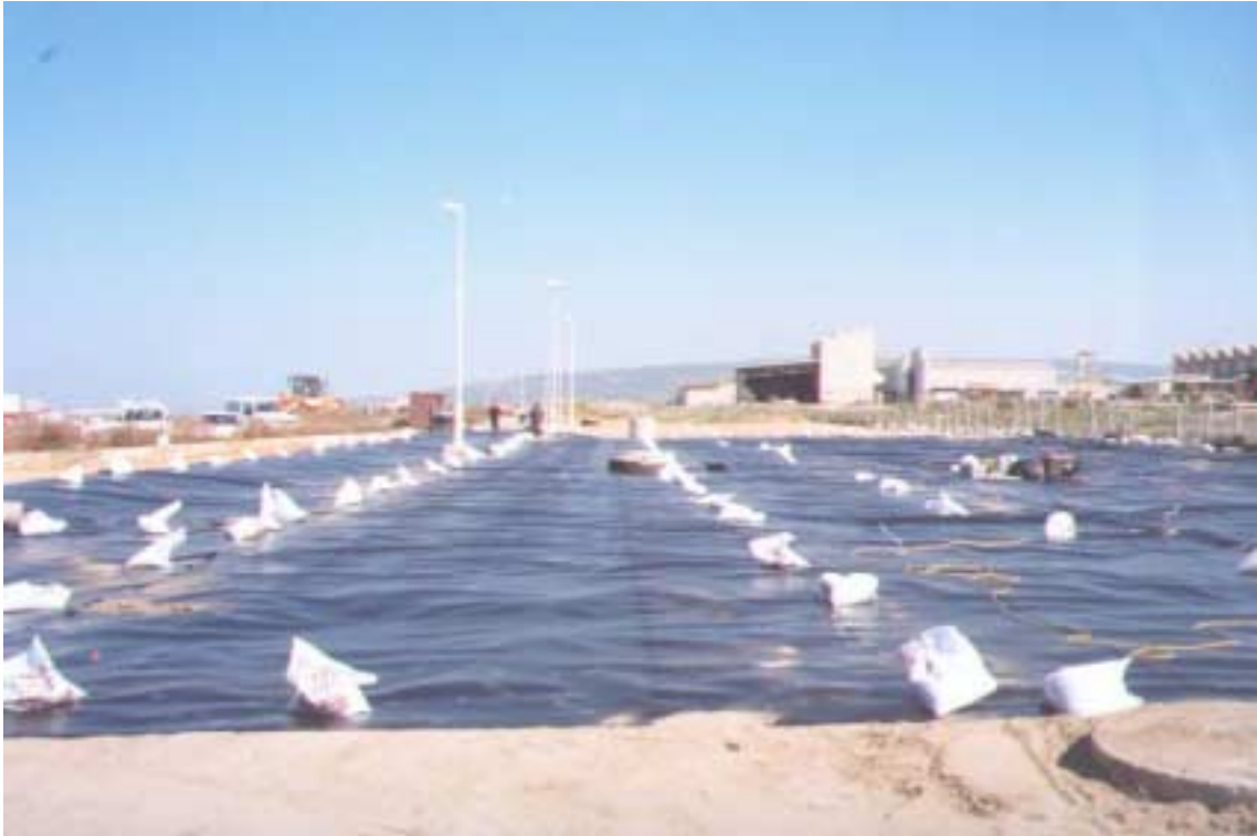
Figure 12. Geomembrane laid out over roadway area. [Full Size]
