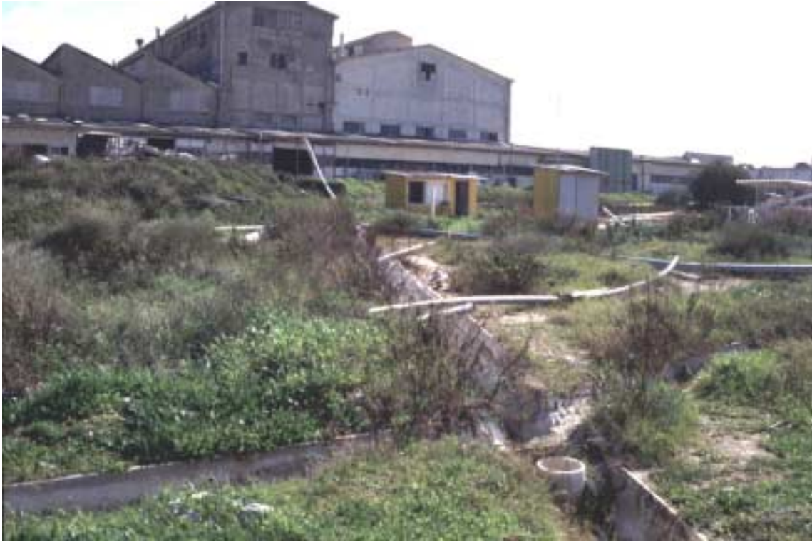
Figure 3. Slurry trenches running downhill from plant. [Full Size]
