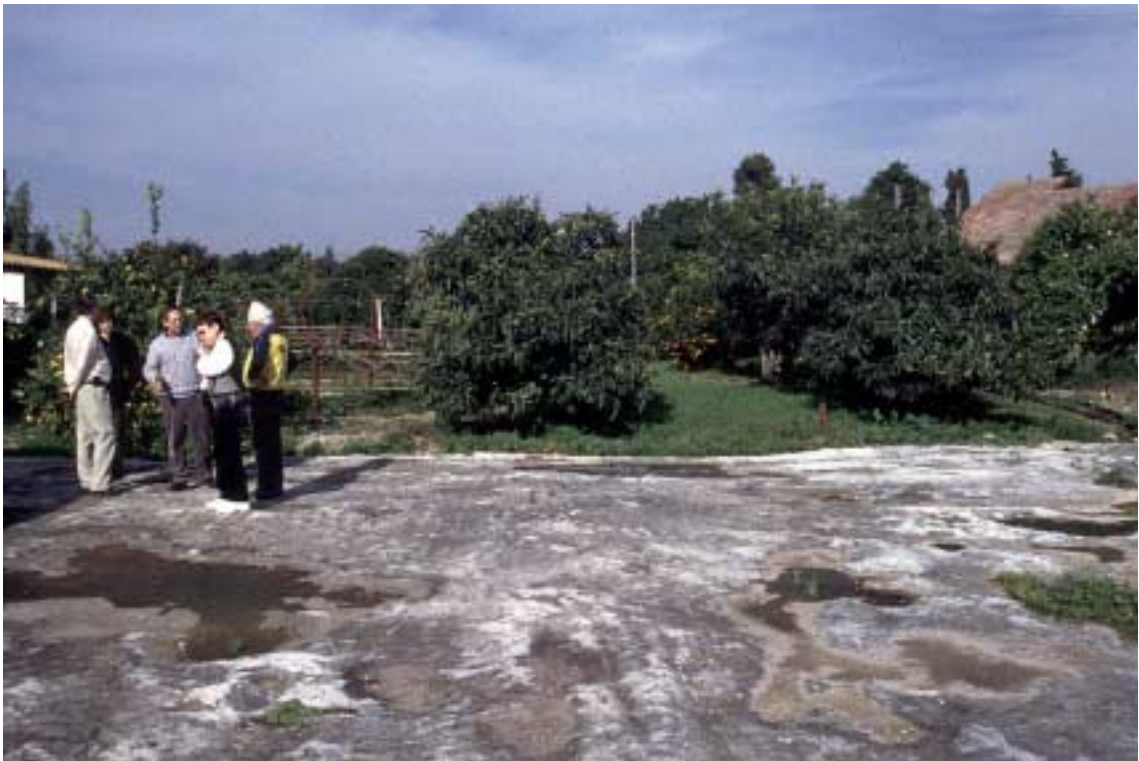
Figure 4. "Cowyard" pavement made from asbestos-cement pipe waste. [Full Size]
