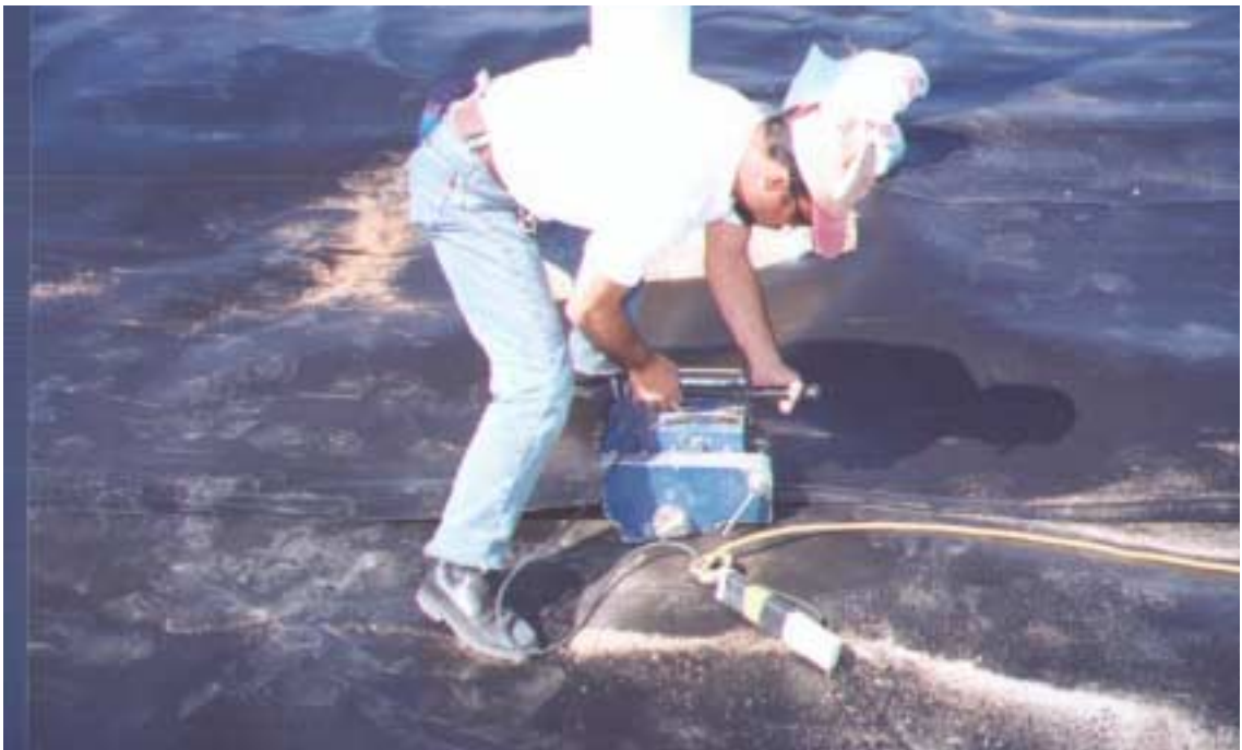
Figure 13. Heat-sealing seams of geomembrane. [Full Size]
