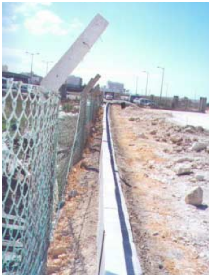
Figure 15. Wall along fence to collect contaminated run-off from plant site. [Full Size]
