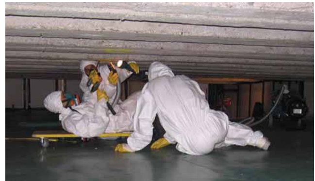
Cramped working conditions
