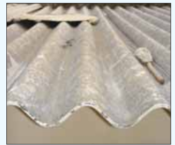
Exterior AC roofing in reasonable condition. Note surface weathering.
